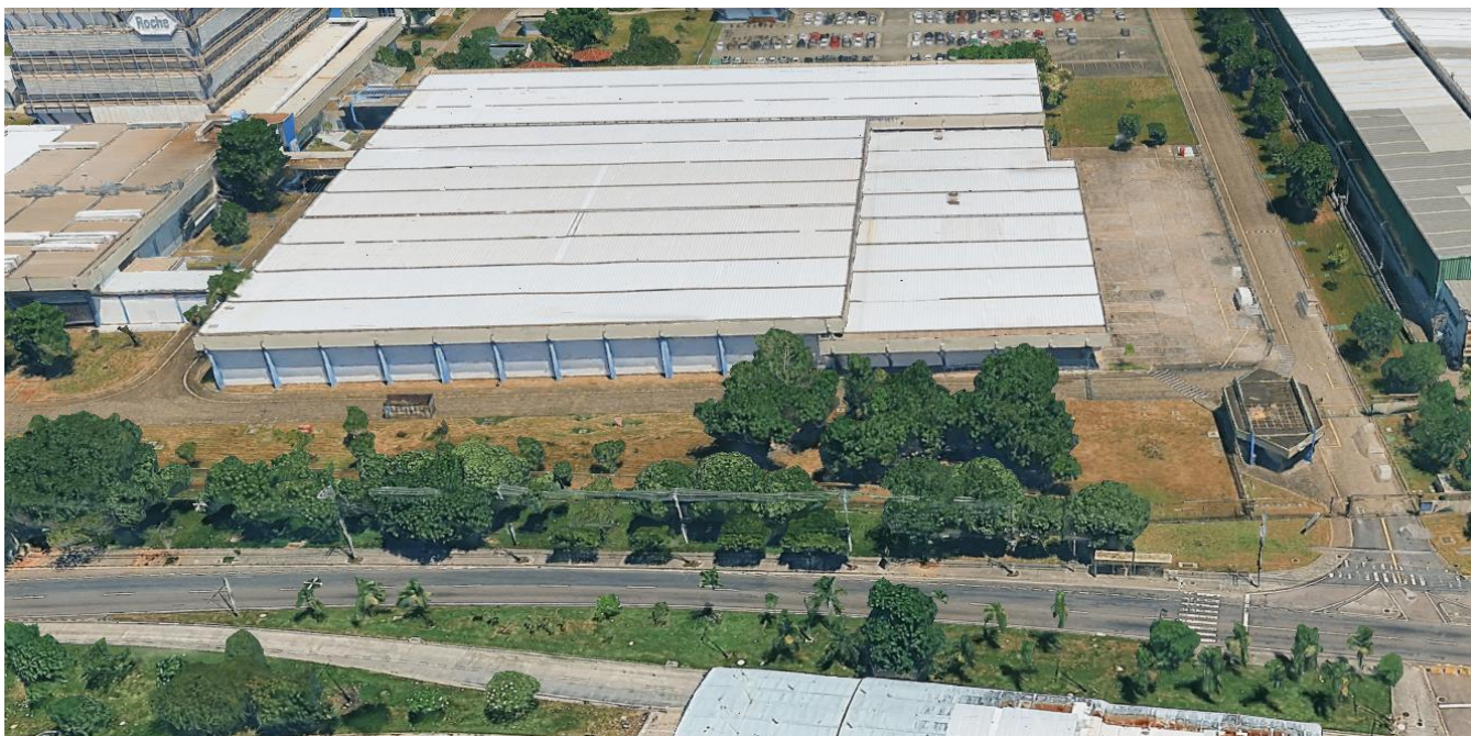
Figura 1 – Fachada Bloco Frontal (Google Maps)
